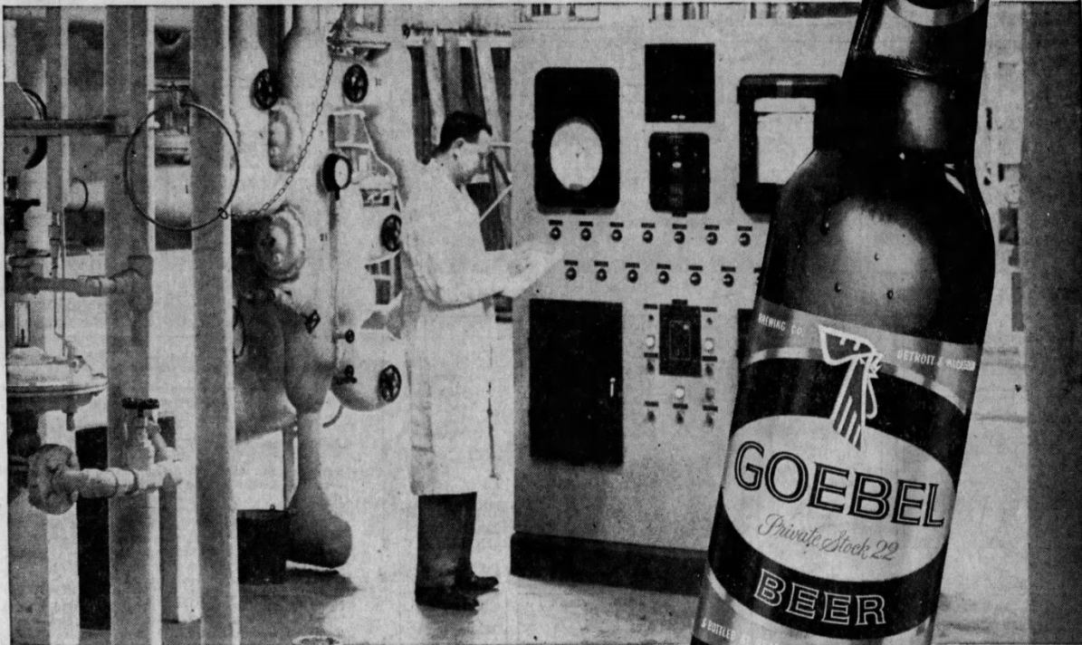
Shown here is the patented Crystilling equipment recently installed at the Goebel Brewing Company. With this installation ordinary city water is made purer than the finest mountain spring water . . . water that is purer than nature's best.
